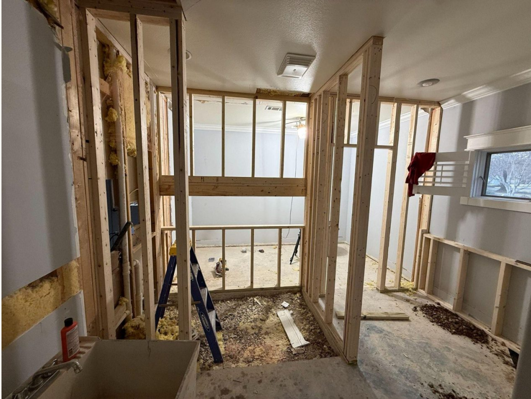
Interior framing during construction
