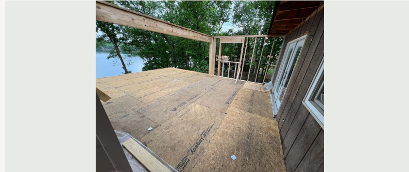
Deck construction progress
