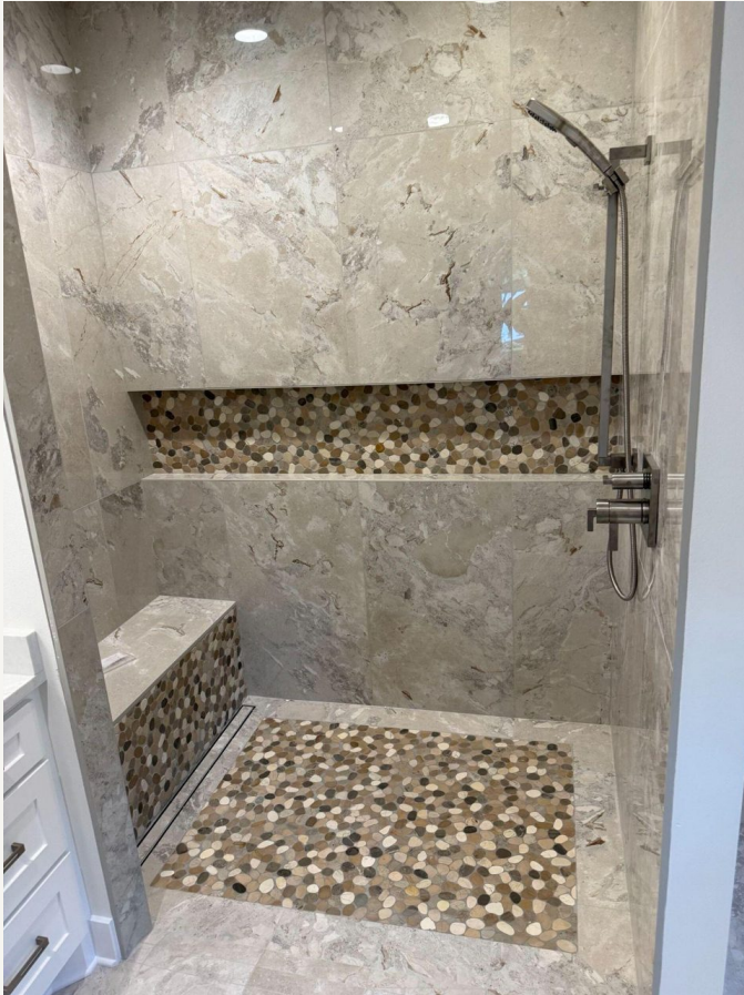
Primary shower: wall and mosaic tile
