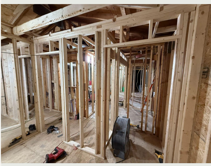
Interior wall framing
