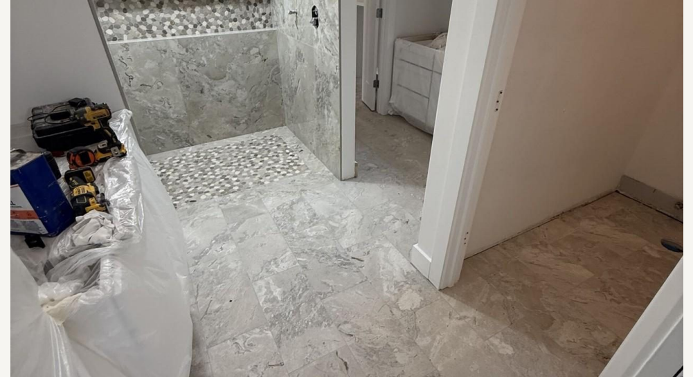
Shower threshold and adjacent floor tile
