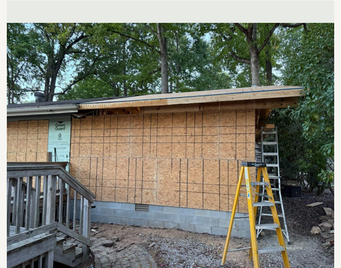
Exterior addition progress
