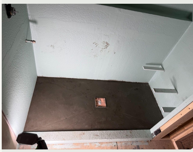
Interior construction progress
