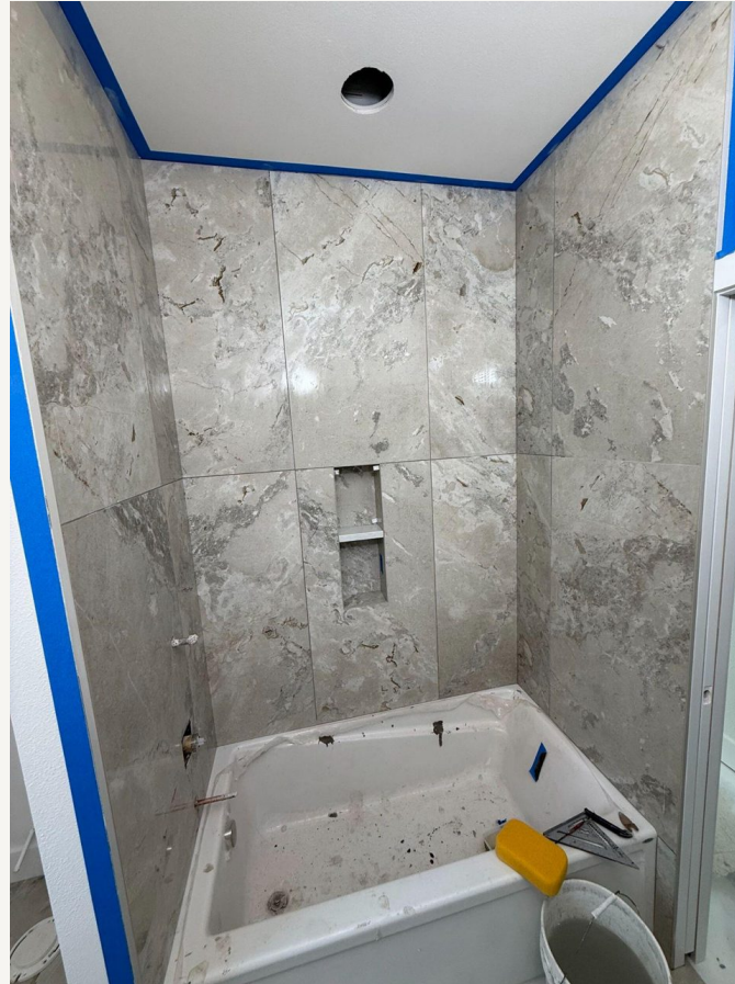
Guest bathroom: tub surround
