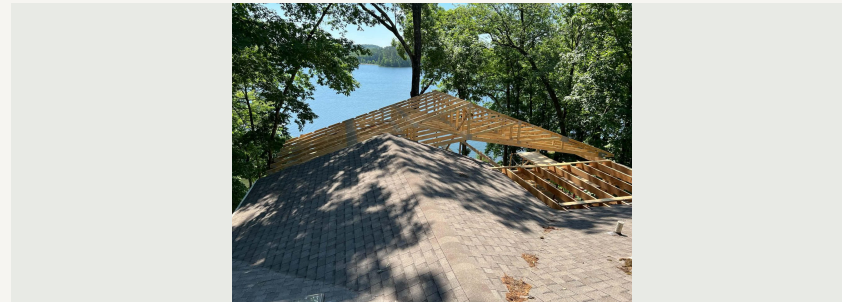
Roof framing progress
